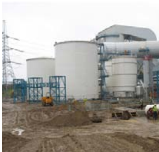
Construction of CCPIlot100+ post-combustion capture project at Ferrybridge, Yorkshire
